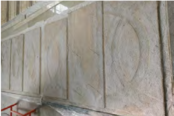
9. Leveling the pattern by net and sand
